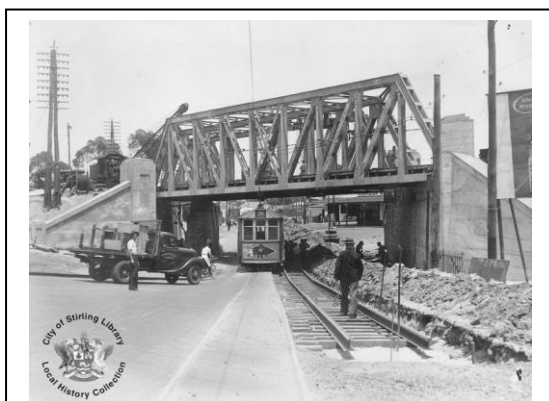
After widening the subway, the 2 nd tramline was laid. Courtesy of City of Stirling Library, Local studies Collection
