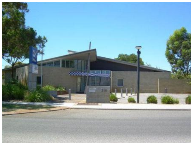
Recent front view of Morley Police Station
