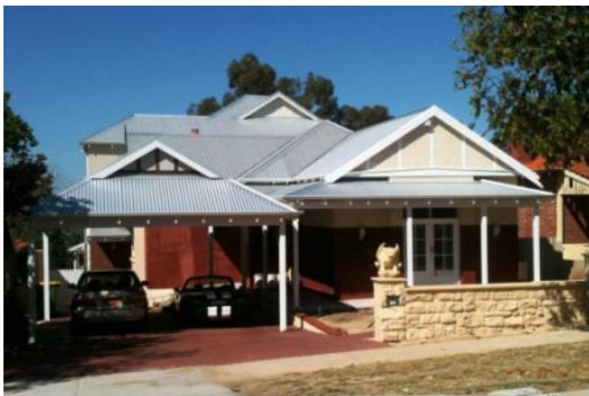
Almost completed; tuckpointing still needs to be finished
