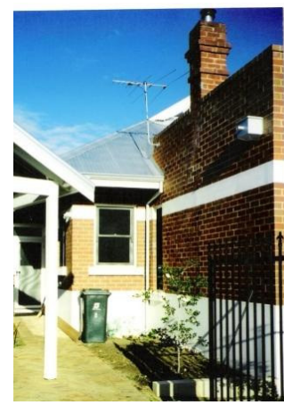
Parapet old and new
