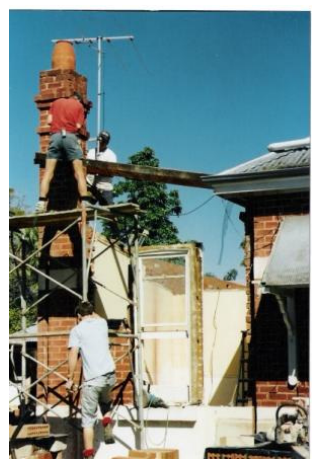
Kitchen pushed out to North ,keep chimney winter 2002
