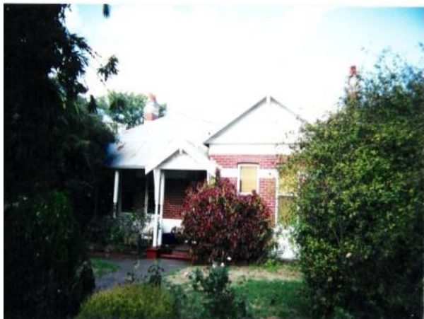
Moorabool prior to renovations
