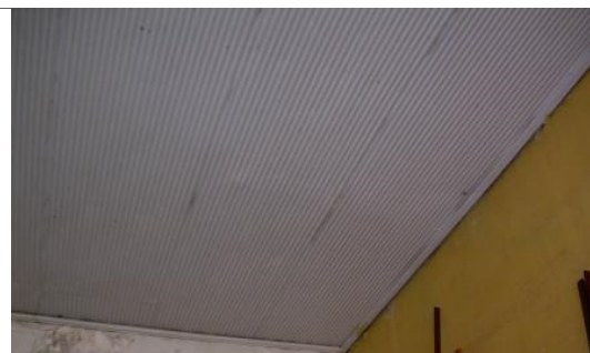
Original ceiling in 159
