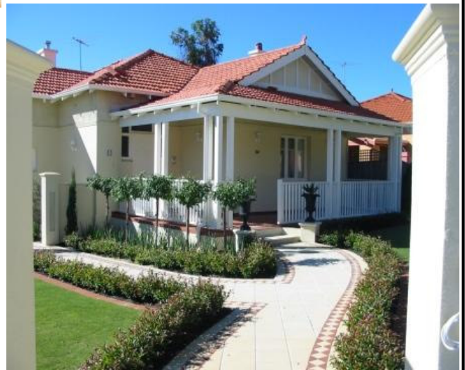
After Renovation Front of house
