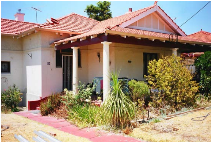
100 Rookwood St Menora prior to renovation
