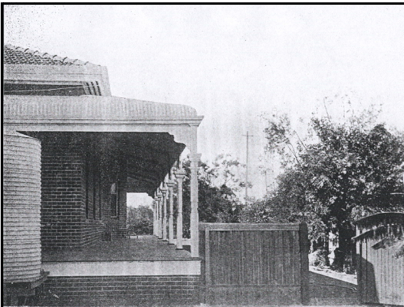
View showing Side Verandah.
