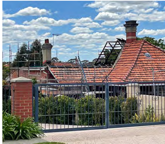
34 Second Avenue Mt Lawley - a repair in progress
