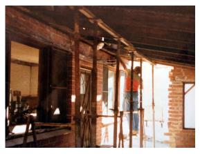
When the final brickwork was done, the tile roof was put on (above left). However, and to make life more interesting, to be able to live in the house while it was being constructed, the rear double wall had to be demolished only after the roof, doors, windows were all in place (above right).
