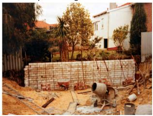
intervals and then dig out a section of dirt and place horizontal planks behind and in between the poles. As I dug deeper, I added planks on top of each
