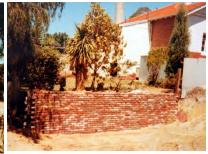
With the actual construction of the addition, the first part of the project was to remove the old laundry and steps to the backyard, break up the concrete and dig out the dirt to the level of the prescribed lower foundation. This took about 22 truckloads of dirt. Then I had to remove the remaining dirt by hand to build the afore mentioned retaining wall (see photos above).
