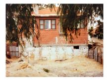
At the same time, a support wall was built to hold up the original back of the house. This was accomplished by building brick columns, one at a time, then filling in between to create one large wall.
