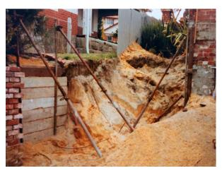
other, until they built a wall of planks. Unfortunately, I had misjudged the depth of one section, and as I reached the bottom area, one of the poles slipped, due to the pressure of the dirt, and the whole lot caved in on me. I was covered in sand to nearly shoulder height and was unable to move. I screamed for help, but no one came to my aid. The neighbours had gone on holiday, so weren't there to
